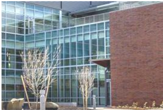
Photo 2: Lower Columbia College Health and Science Building
