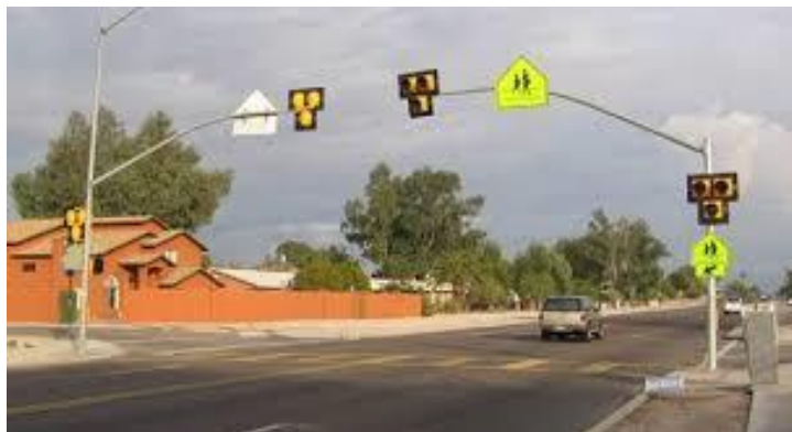
Photo 6: Pedestrian Beacon HAWK (High Intensity Activated crosswalk) in the City of Wenatchee
